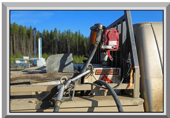
Figure 25.30 Fuel Pump System on Tidy Tank.
