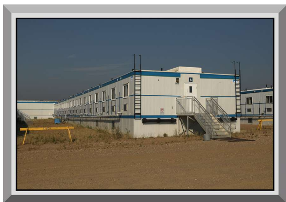
Figure 3.64 Bunkhouse Accommodations in a Semi-Permanent Remote Camp.
